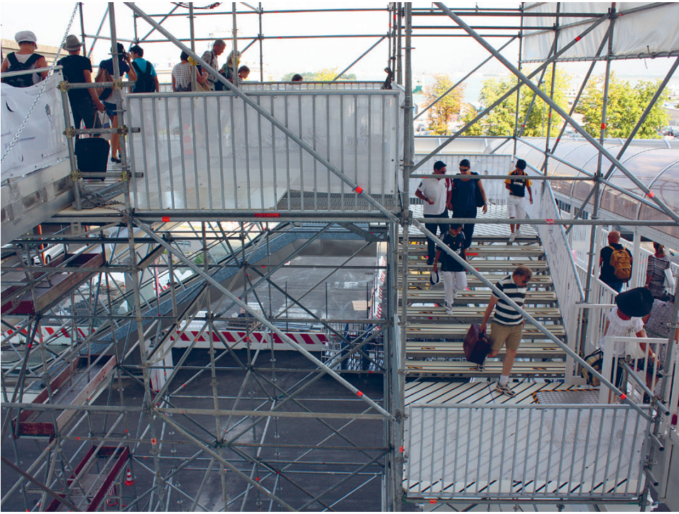
FIGURE 14. Temporary terminal structure in the port of Venice.
