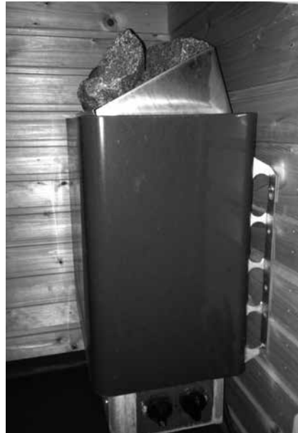
Fig. 4.41. An electric sauna stove.
