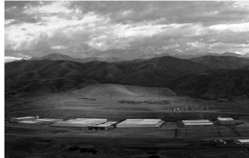
Fig. 1.3. A panoramic view of a remote data centre in Utah that uses up to 1.7 million gallons of water per day available to cool the huge facility (2015). Photograph courtesy of Electronic Frontier Foundation.
