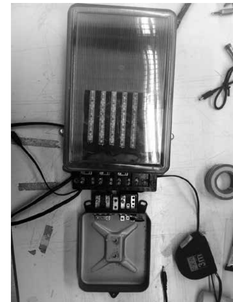
Fig. 4.I5. Rewiring two obsolete electric meters together.
