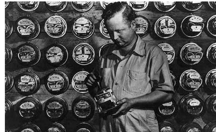
Fig. 4.4. Top , Electrification in progress. Rural Electrification Administration (REA) erects telephone lines in rural areas. Photograph courtesy of National Archives and Records Administration; bottom , Rural electrification in the U.S. Original caption: "This collection of electric meters, receiving a final adjustment, is ready to be installed in U.S. farms where electric light and power have been secured through farmers' cooperative groups. These meters tell how much electricity is consumed each month. Each farmer's cooperative group, operating on a non-profit basis, tries to provide low cost electric service to its members. Such is the trust that the cooperatives have in their members that the members usually read their own meters and sometimes compute their own bills." 16 Photograph courtesy of Library of Congress.
