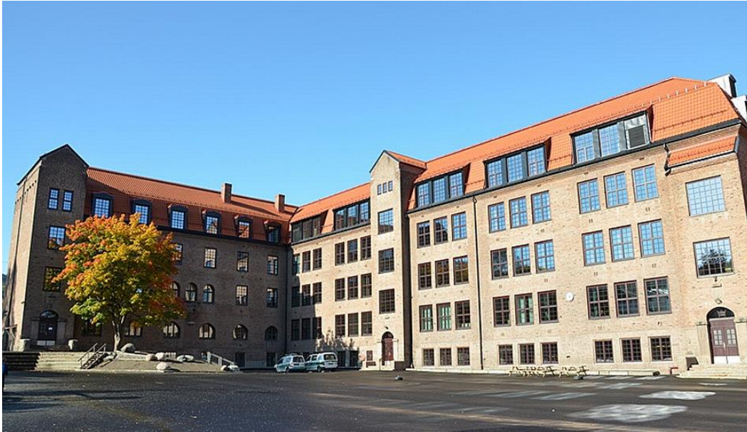
Figure 8. Brandengen school in Drammen, Norway. Photo: www.veidekke.no
