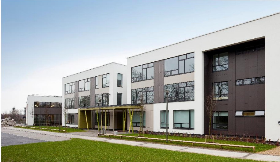
Figure 7. Coláiste Choilm post-primary school in Tullamore, Ireland. Photo: Donal Murphy.
