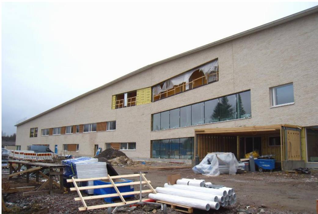
Figure 22. Vehmainen school and day-care centre construction site photographed 9.4.2016. Photo: Paula Sankelo
