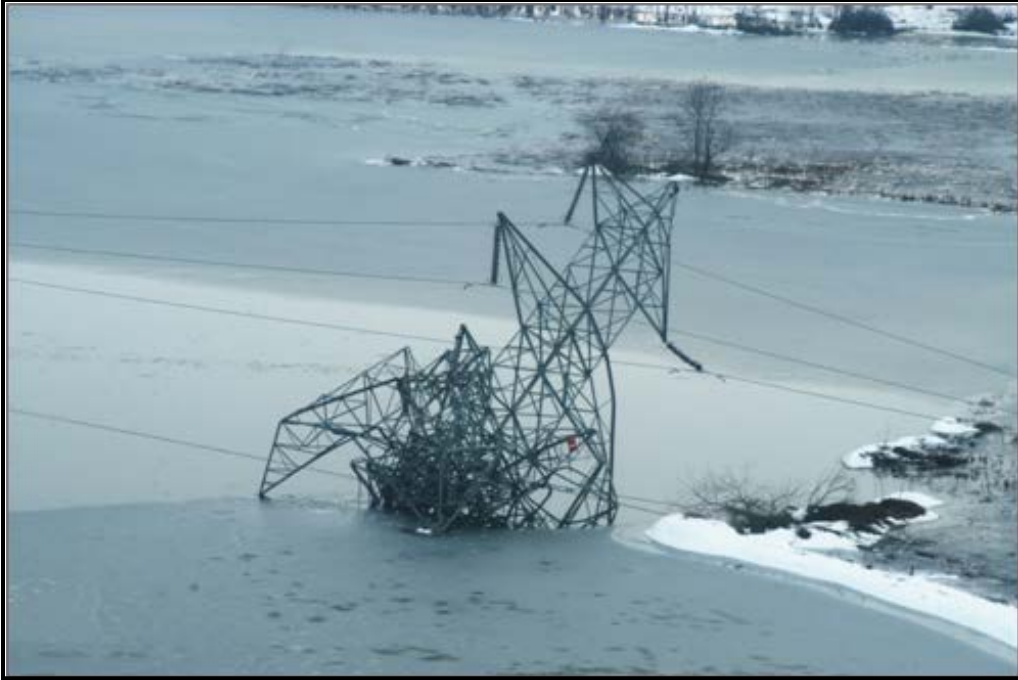
Figure 4.22 Tower Failure caused by harsh weather condition -1 [19]
