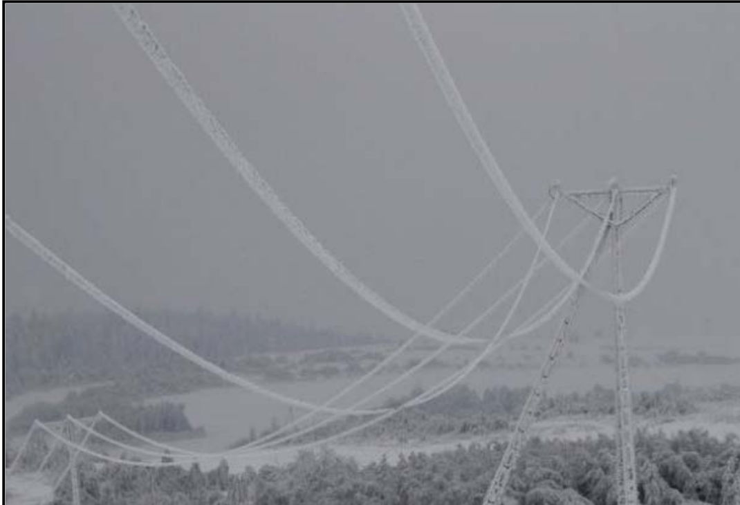
Figure 4.14 Heavily ice - loaded Tower [30]
