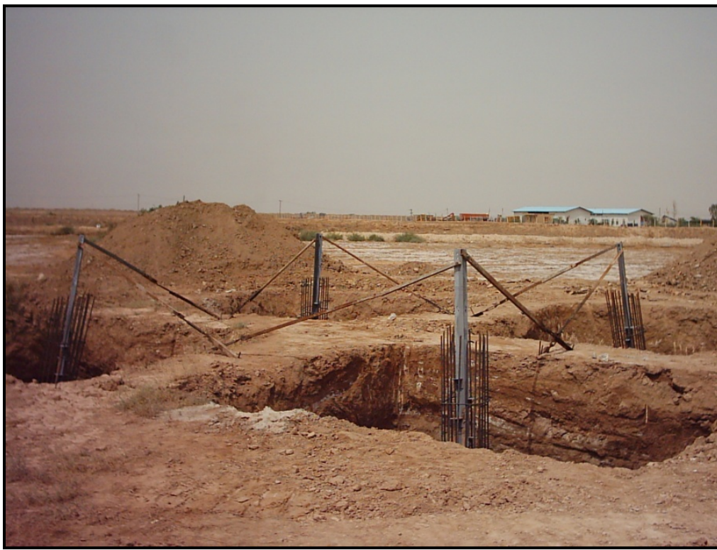
Figure 2.5 Execution of Foundation -1 [19]
