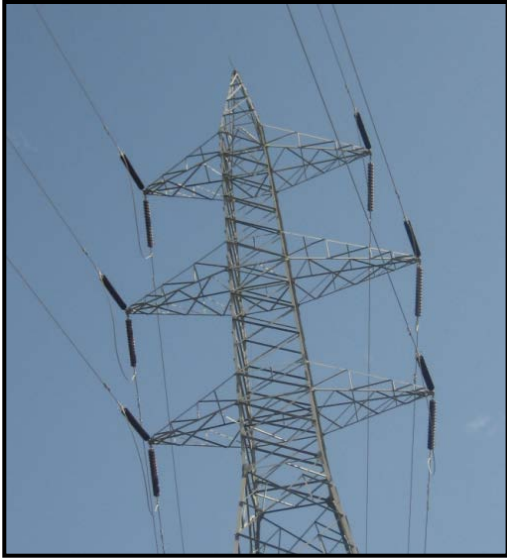
Figure 4.12 Line Angle bisected by Tension Tower [19]
