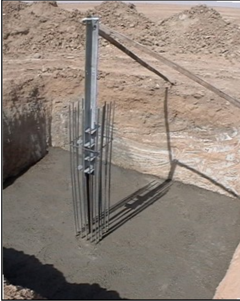
Figure 2.6 Execution of Foundation -2 [19]
