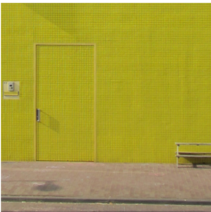
FIGURE 21. STEIGEREILAND, IJBURG, AMSTERDAM, NETHERLANDS.
