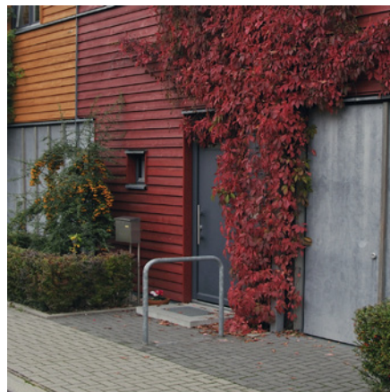
FIGURE 34. TOWNHOUSE, ROSSMÄSSLERSTRASSE, LEIPZIG, GERMANY.
