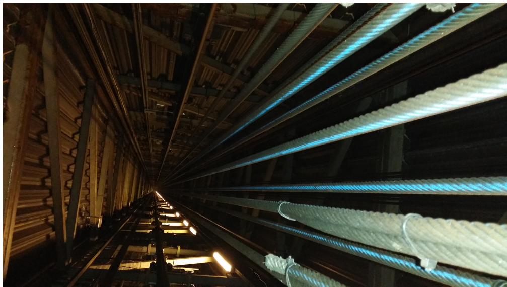
Figure 28: The steel shaft and ropes of Tytyri.
