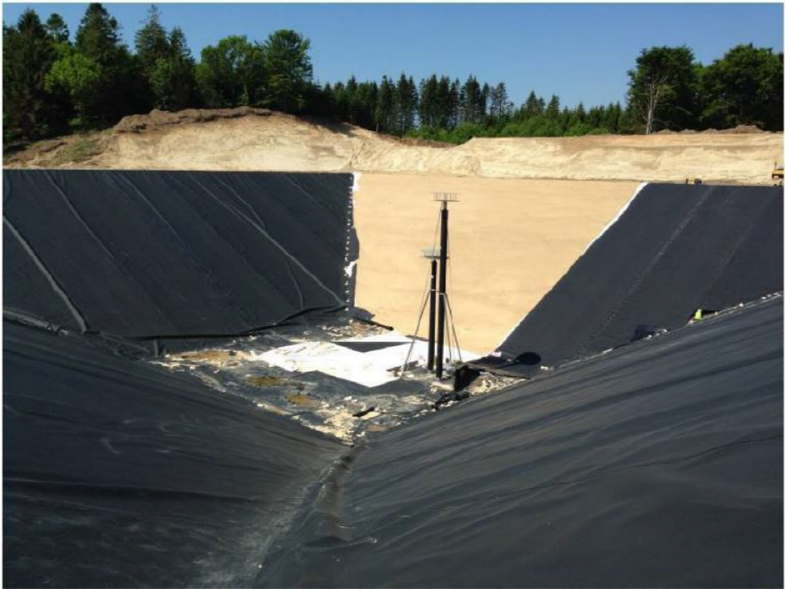
Figure 26: Excavated slopes at SUNSTORE 3 storage in Dronninglund. (Jensen, 2014)
