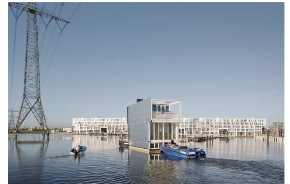
Figure 11. One floating module house going to the site.
