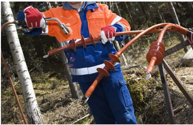
Figure 8: Heat-shrink termination installed onto a 20 kV three-core cable [14]
