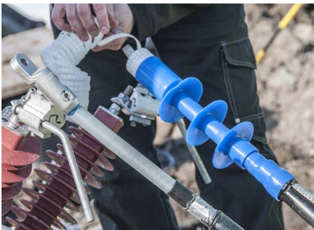
Figure 9: Pre-stretched cold-shrink termination installed onto extruded 20 kV cables [15]
