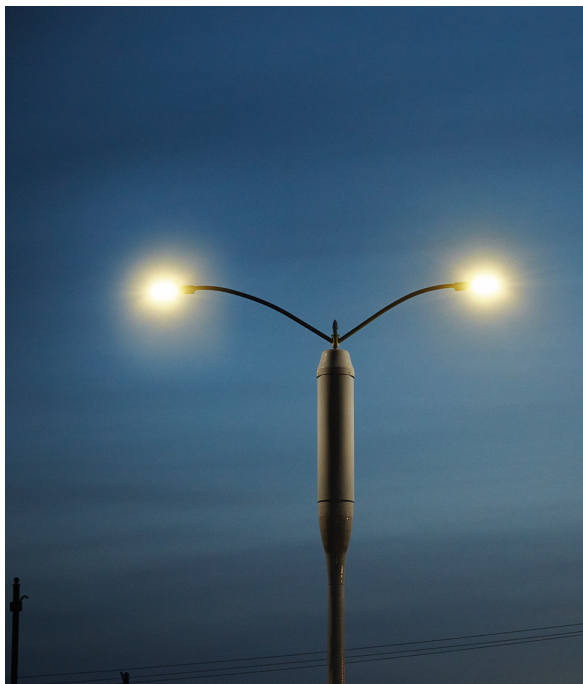
Figure 14: Zero site concept released together by Ericsson and Philips. The thick part of the pole contains base station hardware and antennas. [47]
