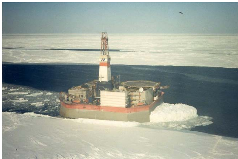
Figure 4: The Molikpaq is an octagonal mobile caisson that was used for oil exploration in the Canadian Beaufort Sea. The data collected from it has been widely used in ice mechanics research (Sudom and Timco, 2009).
