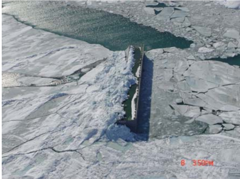
Figure 3: Ice barriers are wide structures that are often built in shallow water to protect offshore structures and ports from moving ice. The ice is pushed against the structure from the left and a large amount of rubble has formed in front of the structure. Furthermore, there has been overtopping as some ice has ridden on top of the ice barrier (Croasdale et al. , 2011).
