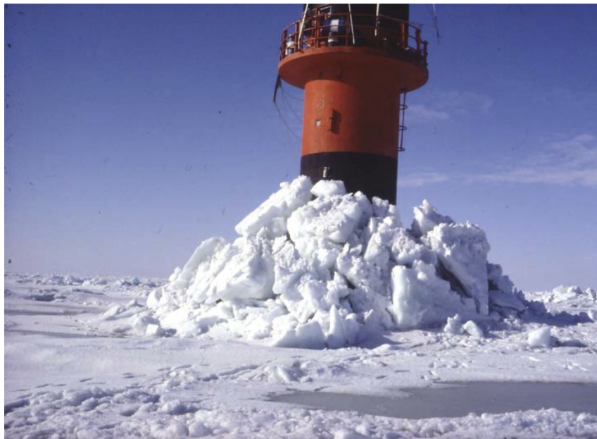
Figure 1: Arctic offshore structures are subject to ice loads when the ice interacts with the structure. A large ice rubble pile has formed in front of Kemi I lighthouse as the advancing ice has failed against the it. The image shows the sail of the pile while the rest of the rubble is under water. (Image by the courtesy of Mauri Määttänen.)
