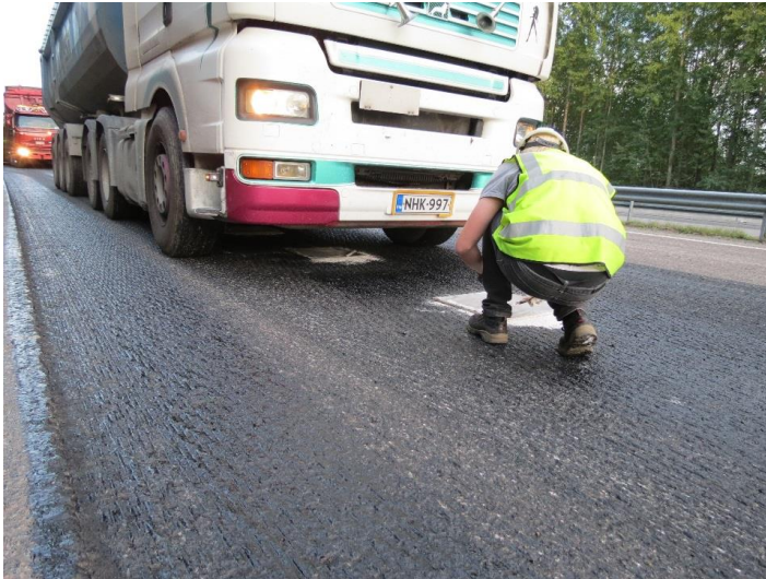
Figure 31. Placing more grease on the wooden plates.
