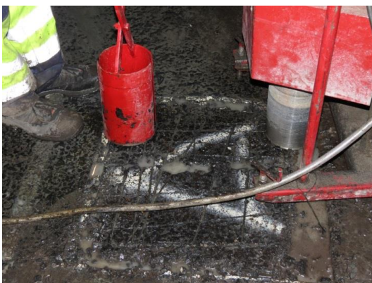
Figure 28. Cuts made in the slab to remove the mixture.
