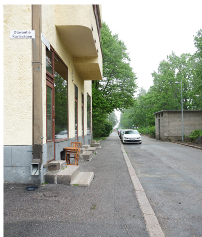
Figure 3 Narrow pavements with cross-fall and entrance steps are felt unsafe.
