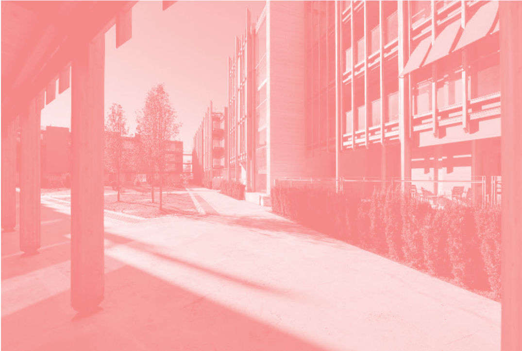
Common spaces between buildings
