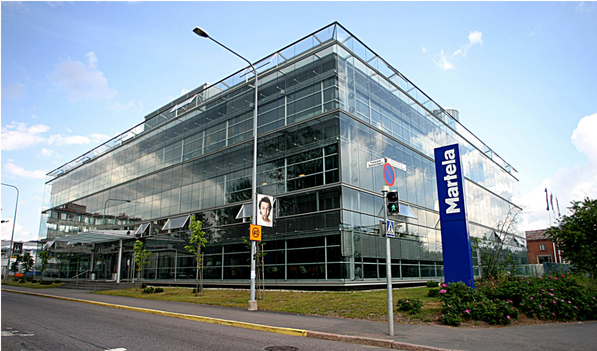
Figure 18 Photograph of the Martela Business Center
