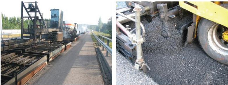
Figure 3. Hot in-place recycling: heating, milling and addition of new fresh mixture.
