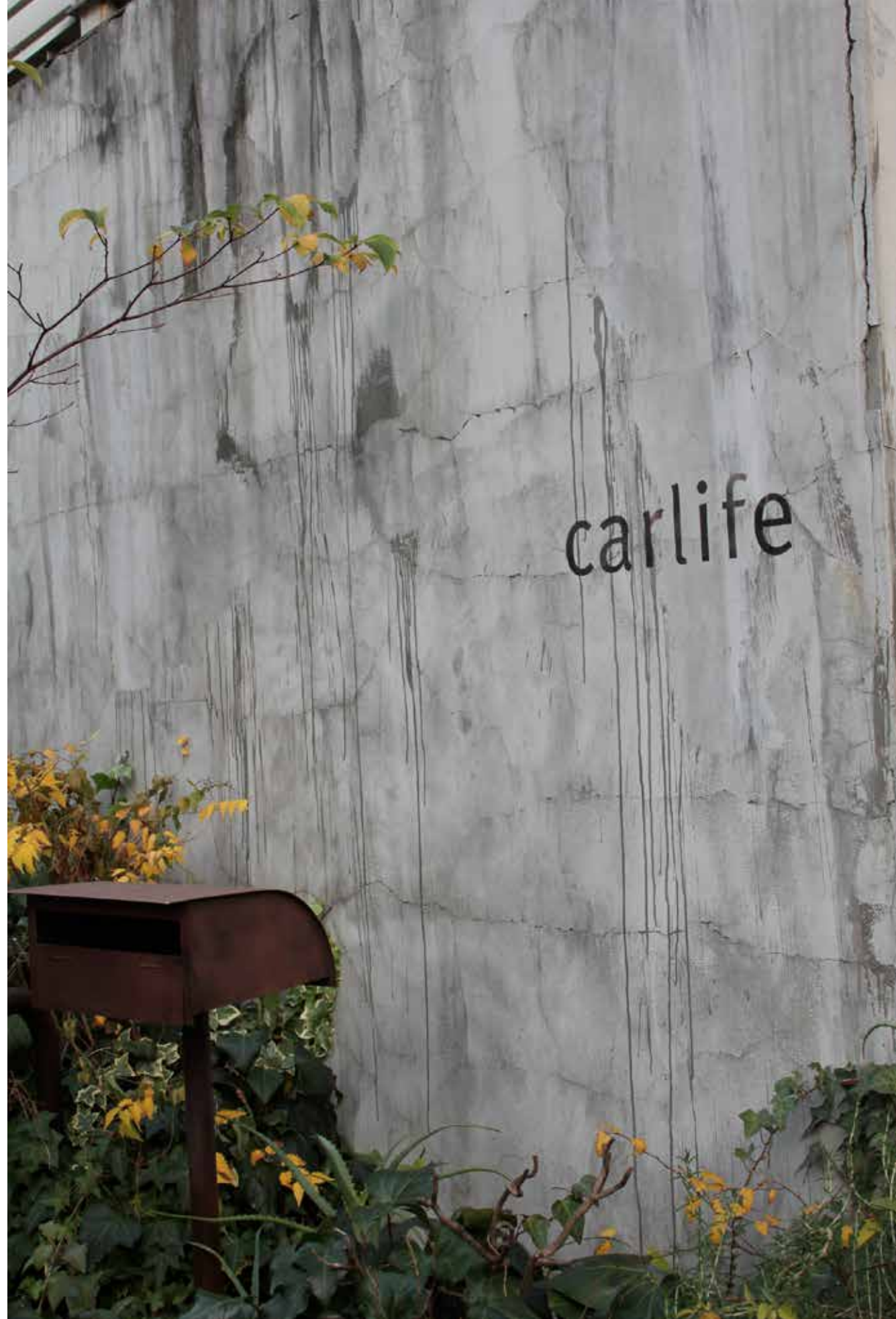
Picture 97. Facade in Naga-Meguro, Tokyo.
