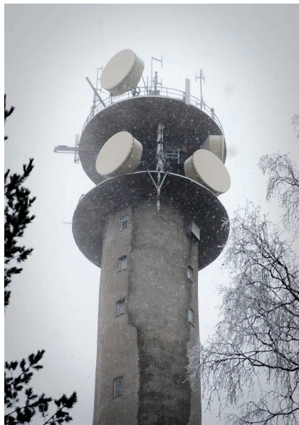
Figure 45. The program distribution radio link networks, operated by Digita on 3.6 - 4.2 GHz. The connections are partly analogue, partly digital. Link span lengths are on average less than 100 km.
