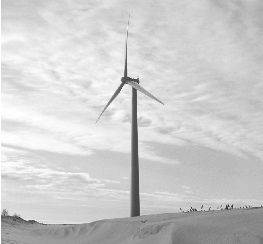
Figure 2. Three-bladed horizontal axis wind turbine with 1MW nominal power, courtesy of WinWinD.
