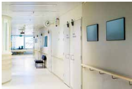
After the renovation at the surgery ward where the pilot project was carried out.
