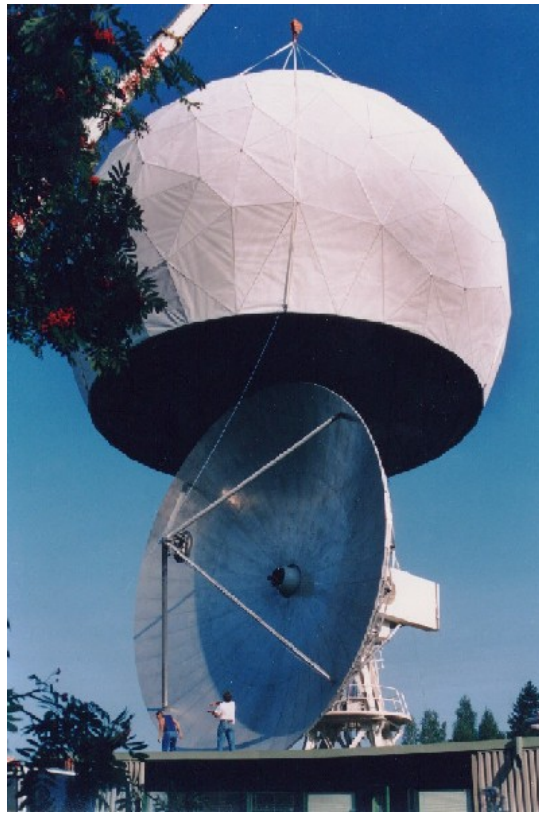
Figure 2.2: 14 m Cassegrain telescope in Metsähovi Radio Observatory.
