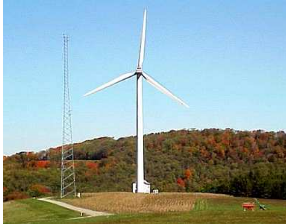
Figure 9: Wind Power turbine deployed at BS
