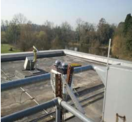
Figure 2-3: Bayfordbury, East of England Science Learning Centre roof.
