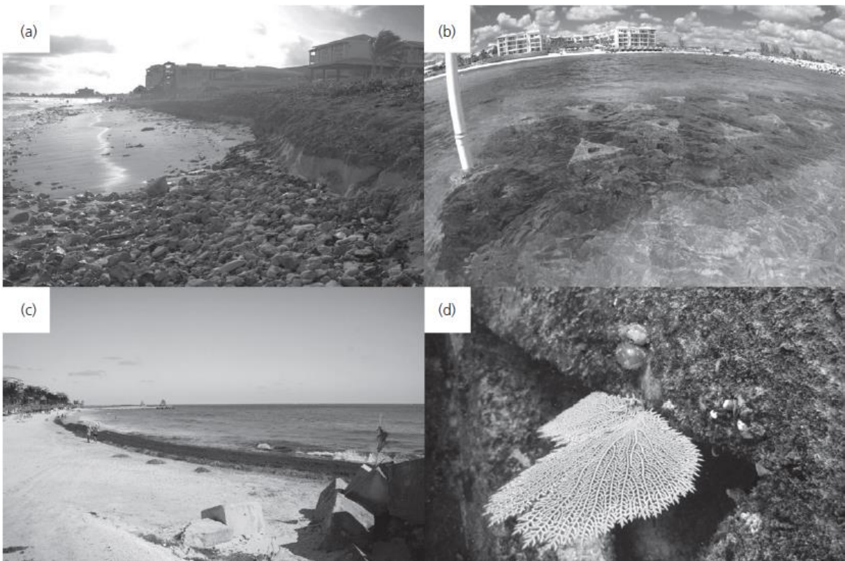
Figure 5. An artificial reef improves coastal protection. (a) Erosion in hotel grounds, (b) prefabricated concrete structure, (c) seagrass crisis and (d) coral colonies established on the structure after 5 years
