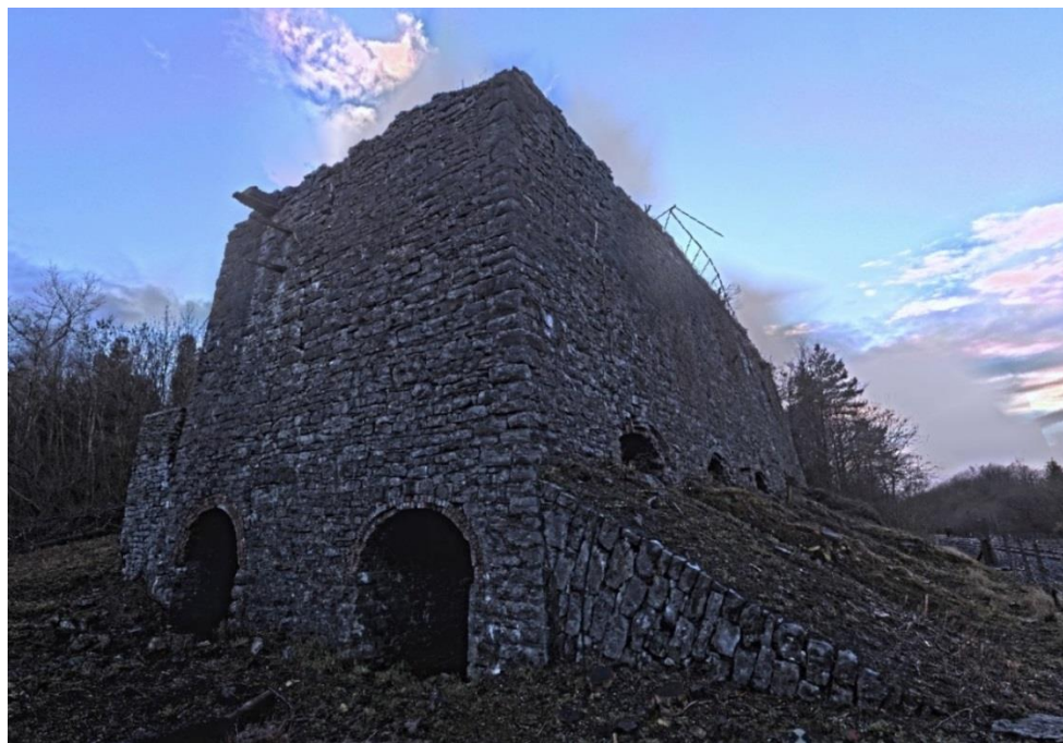
Figure 8-2 Bellmanpark Limekilns (source: GI-RST)
