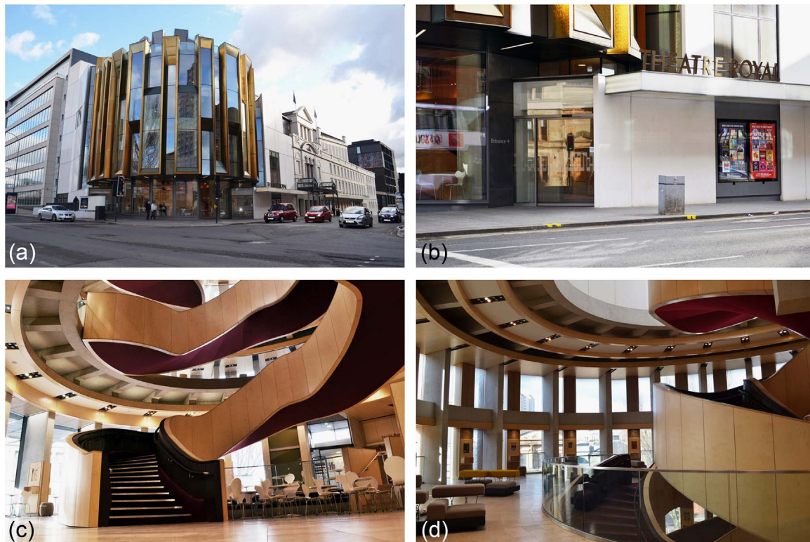
Fig. 2 Theatre Royal (Source: L. Maclean) (a) external view, (b) entrance, (c) staircase, (d) first floor.
