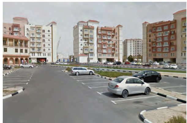
Figure 8. The built environment in the back of main roads in Dubai International City (Source: Authors).
