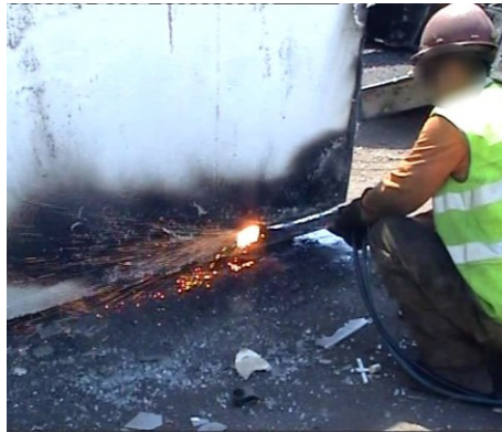
Figure 6: Torch Cutter in the Secondary Zone
