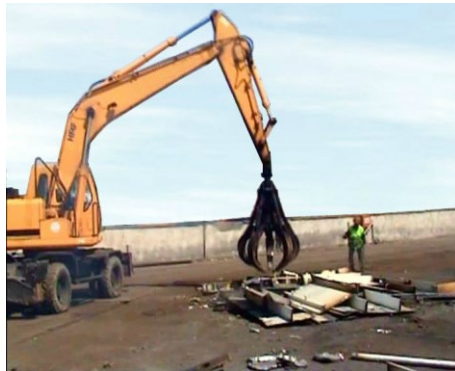
Figure 7: Poly-Grab Crane in the Secondary Zone
