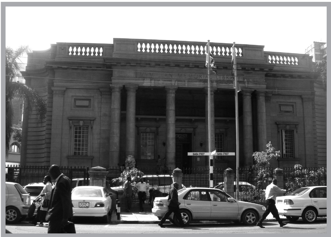
Fig 4. McMillan Library, Nairobi, completed 1931, designed by John Sinclair and Messrs. Rand Overy and Blackburn. Photograph: S. Longair.
