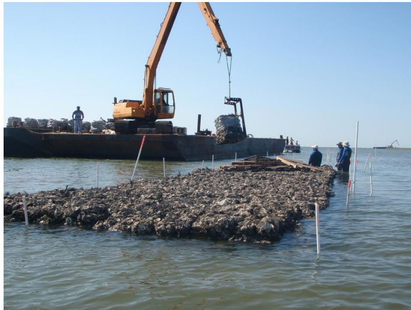
Figure 1.2. Image from NOAA (2015), artificial reef block modules being placed in Alabama, note the second crane in the background showing the scale of the project.
