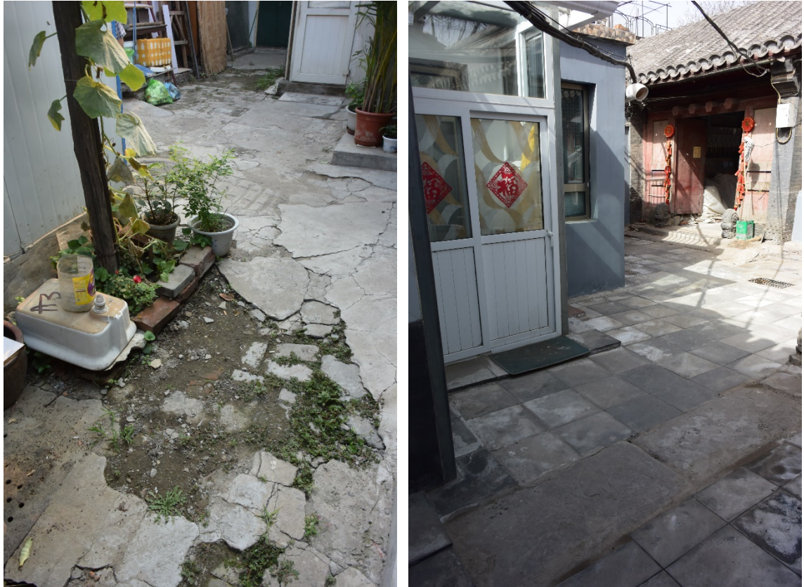
Figure 42. Paving. Before: The seriously destroyed pavement (left); After: The pavement renovated by the SHHPS by using more adaptive materials (right). Photo by Haoyu Wang, Beijing, July 2015 ( left ) and March 2016 ( right ).
