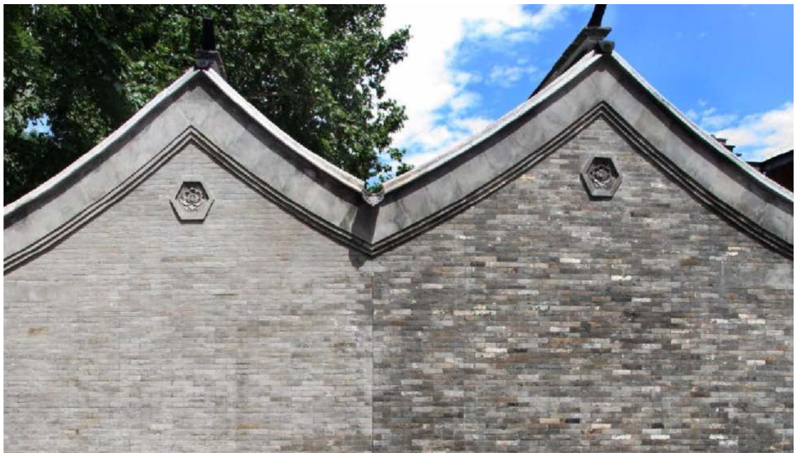
Figure 28. The Garble Wall Are Not the Same Color to Show the One on the Right Was Built Using Old Materials. Photo Source by http://www.princes-foundation.org/what-we-do/projects/cn/shijia-courtyard-24-beijing-china-regeneration
