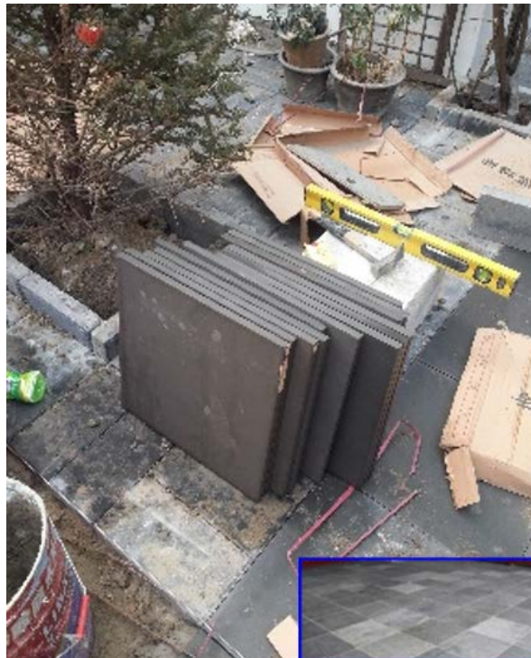
Figure 41. The smaller and thicker archaized paving bricks can better fit and tolerant with the soil (top); The larger but thinner permeable bricks cannot adapt to the courtyard soil in an extreme weather, also it cannot bear the load as heavy as an archaized pavement (bottom). Photo by the Beijing Municipal Institute of City Planning & Design, Hong-Du Design Department, Beijing, November 2015.
