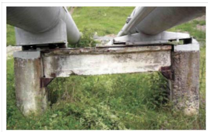
Fig. 5. Overall view of the mounting group of the oil pipeline with the D = 720 mm, whose frame is leaned onto the riser and girder.
