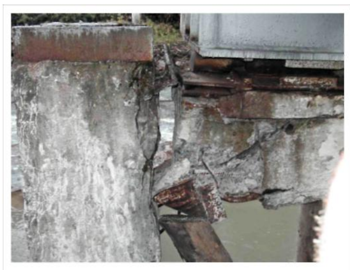
Fig. 2. Destruction of the mounting group of the second oil pipeline support D = 720 mm
