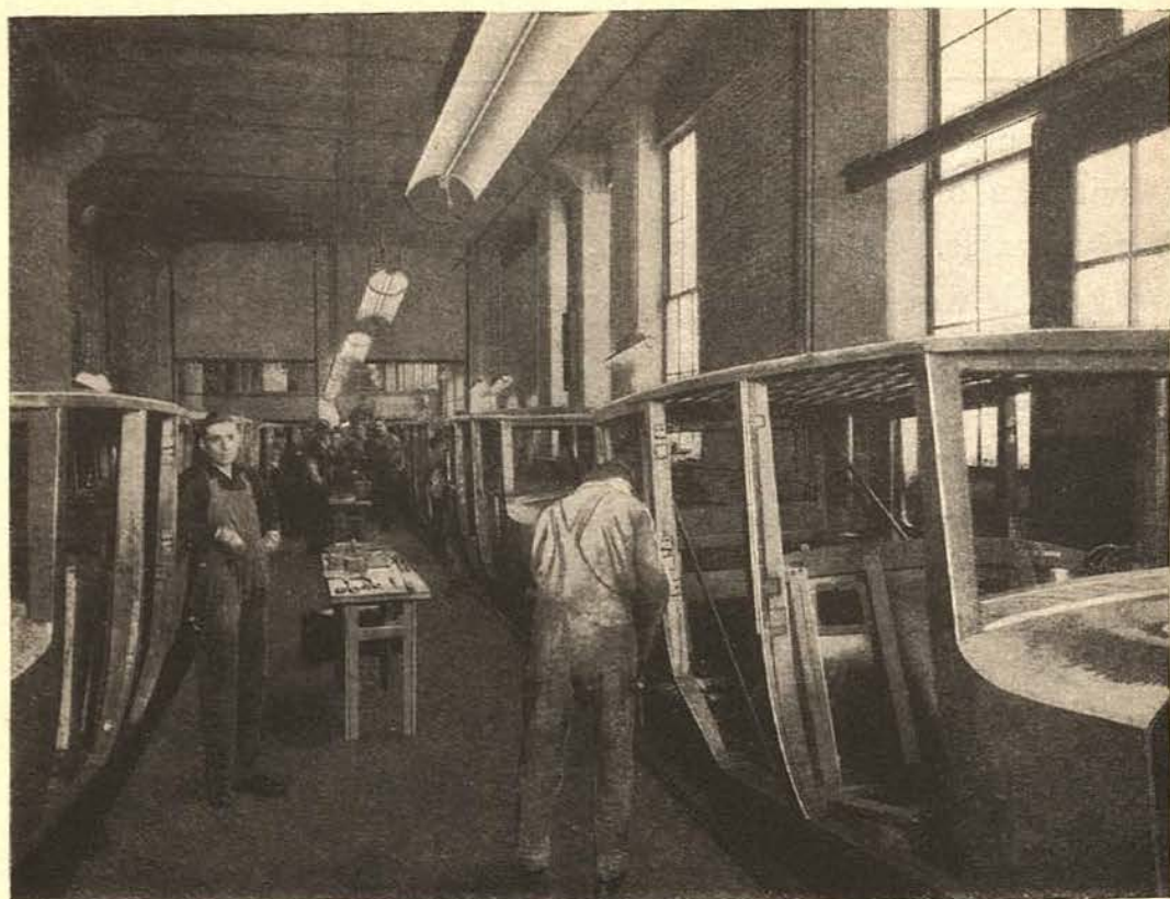
PLANT NO. I, PANELING CLOSED BODIES
