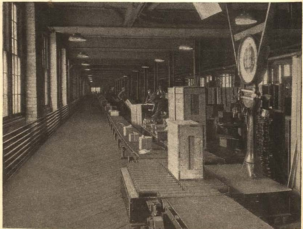
PLANT NO. 5, PARTS SHIPPING ROOM
