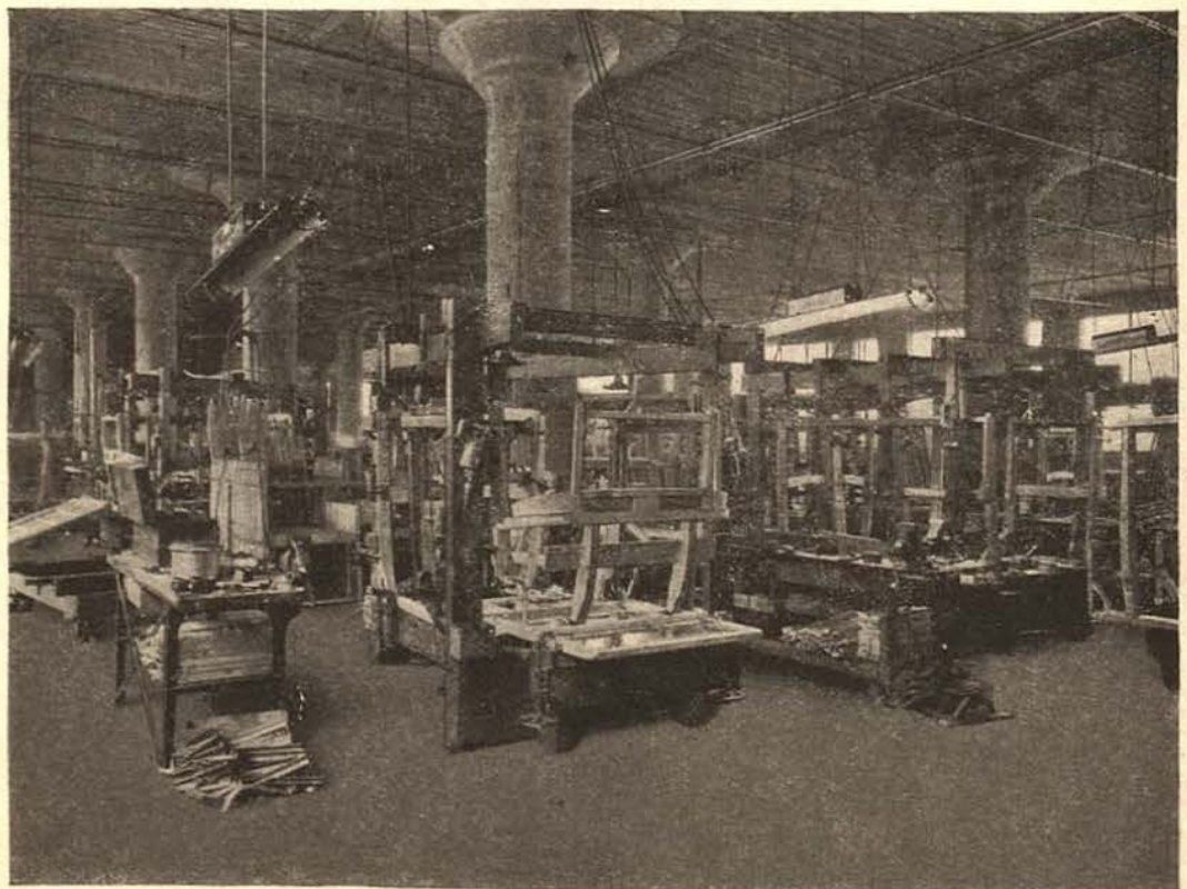
PLANT NO. 1, CLOSED BODY FRAMING
