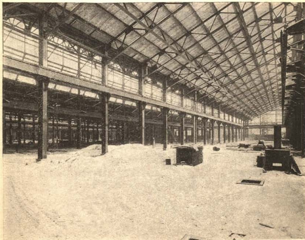
PLANT NO. 2, VIEWS OF NEW IRON FOUNDRY—UNDER CONSTRUCTION
