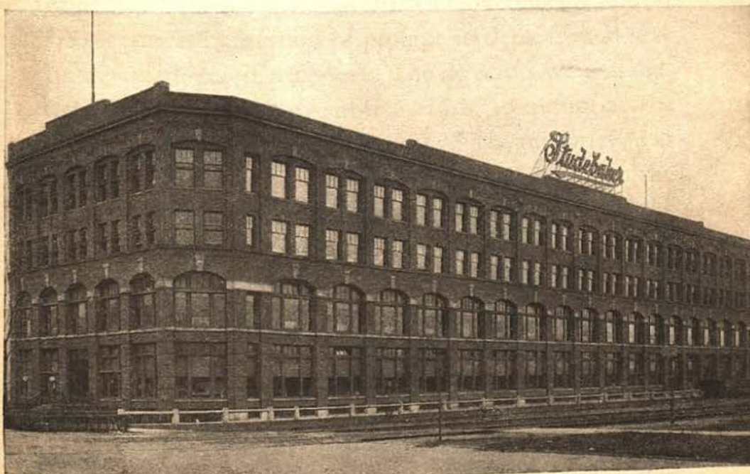
ADMINISTRATION BUILDING, SOUTH BEND, AND INTERIOR VIEWS
