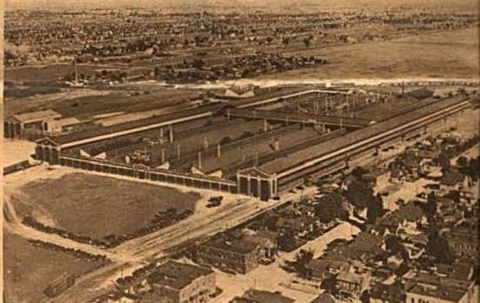
In 1922 Ford of Canada's expanding business demanded more space and Plant 2 was built. It had a total floor area of 640,432 square feet and machine shop operations were moved from the riverfront buildings to the new plant, then classed as one of the largest in the Empire.
