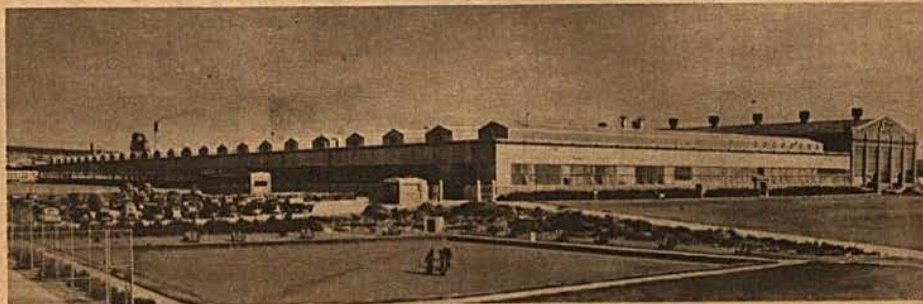
Completed in 1948, the plant of Ford Motor Company of South Africa, Limited at Port Elizabeth is one of the finest and most modern factories in the Commonwealth, and employs almost 1,100 persons. The original South-African plant had been established in 1923.
