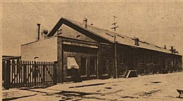
The original plant of Ford of Canada, a former wagon works.
