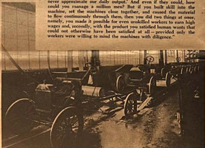
The first chassis assembly line comprised a rope and windlass, the frame being dragged along the floor. This was the first mechanically driven line.
