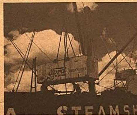
Many vehicles destined for overseas countries are shipped from Ford of Canada's plant in knocked-down condition for assembly abroad.
