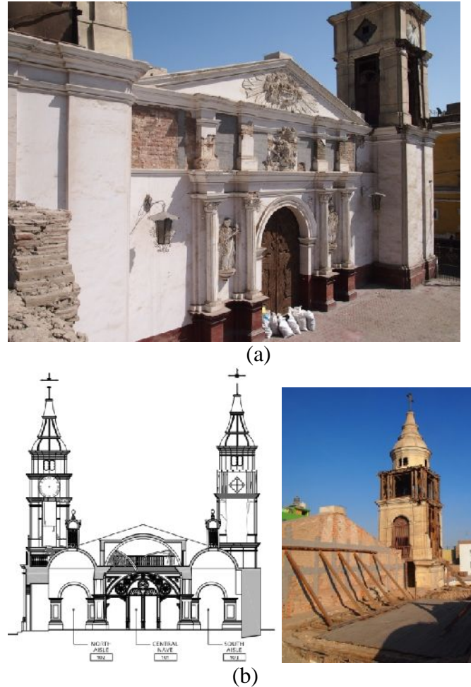
Figure 1. Front façade of the Cathedral of Ica (a); main façade drawing and view of the gable from the back side (b).
