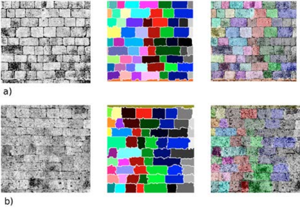
Figure 9 Result of segmentation in two zones of Alçaçova Wall with different image quality.
