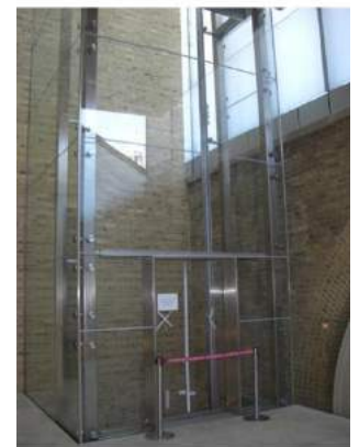
Fig. 50 - Daylit Gallery V&A Museum, London - McInnes Usher McKnight Architects
