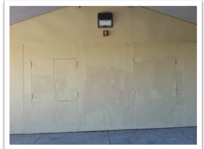
Figure 13: Bathroom After Paint
