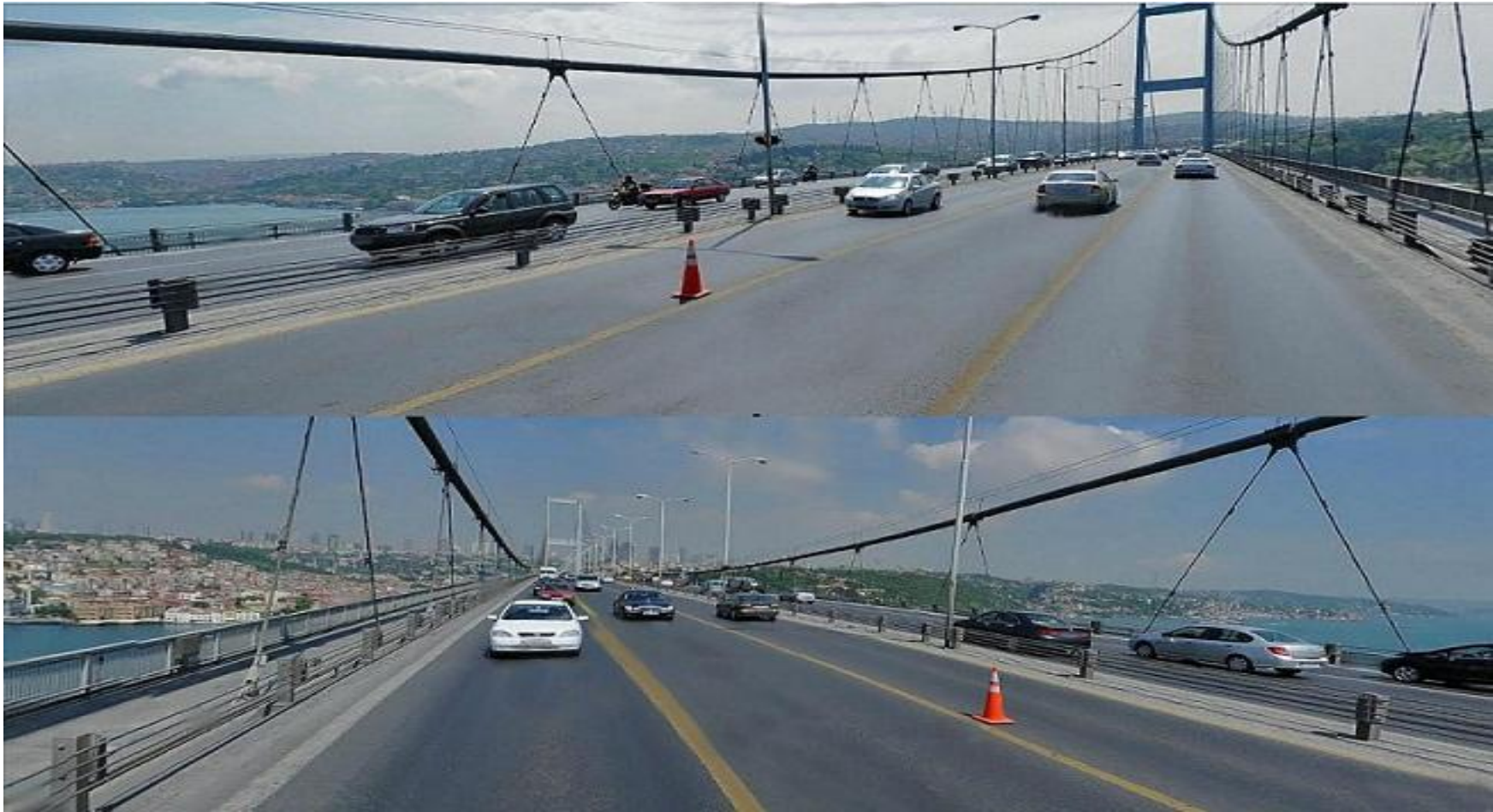
Figure 4.2 : Reversible operation on Bosphorus Bridge.
