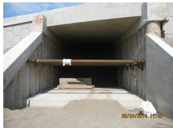
Figure 1: Photograph of Temporary Shoring System
