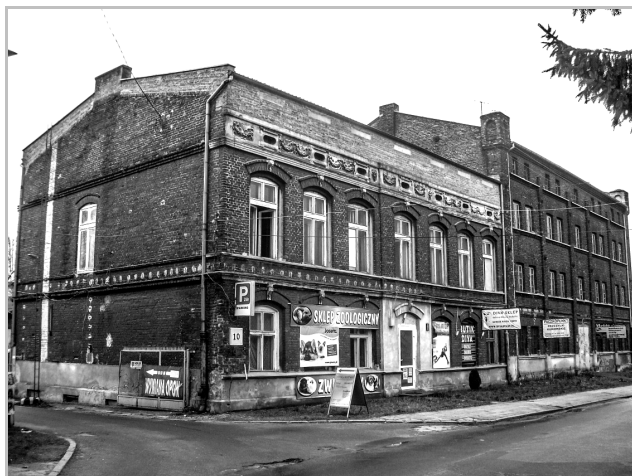
Photo 7. The old mill building 'Rokicie' on Cieszyńska St 10 Photo: P. Moniewski
