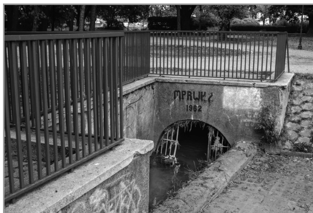
Photo 1. Stormwater overflow by the Jasień in Widzewski Park Photo: J. Jędruszkiewicz
