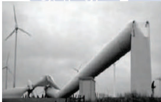
Figure 1.1: Example of catastrophic event: broken wind turbine.
