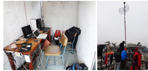
Fig. 3. Server Base (Left) and Main Antenna (Right) in Pokhara City
