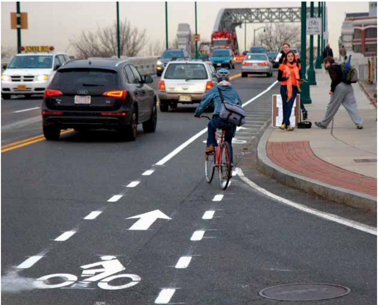
The newly rehabilitated Boston University Bridge features bicycle lanes and other elements of “complete streets” design that facilitate biking and walking. Photo courtesy of Livable Streets.
