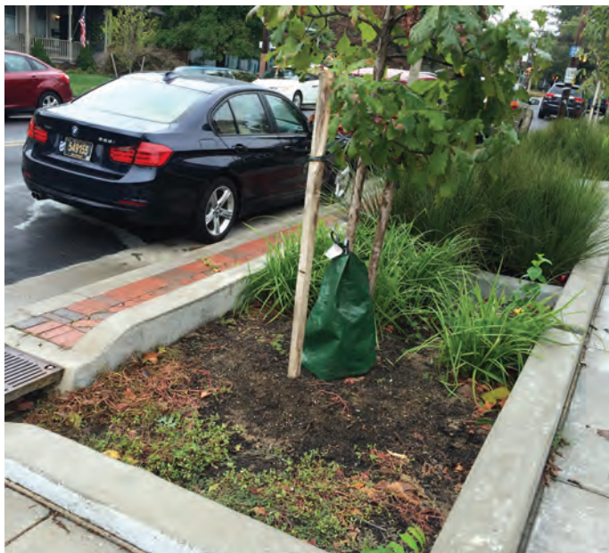
A “stormwater bumpout” like this vegetated curb extension in Washington, DC, expands the available rooting zone for existing trees and significantly slows rainwater runoff during storm events, while slowing traffic in residential neighborhoods.
