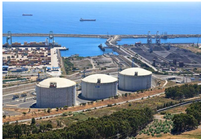
Figura 5.4 - Terminal de GNL de Sines; [REN, 2014a]
