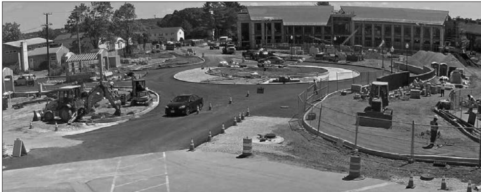
PHOTOS OF HUXLEY AVENUE DURING CONSTRUCTION AND AFTER ITS COMPLETION.
