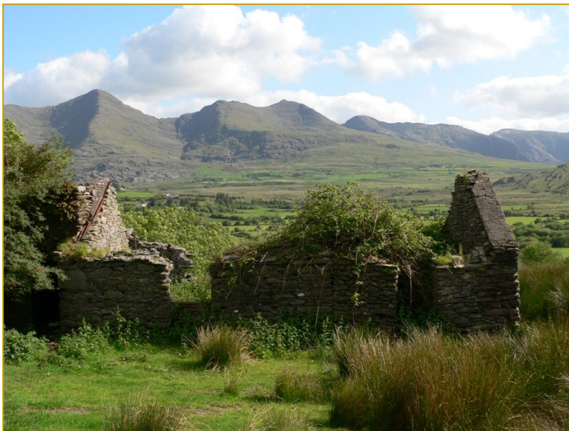
Abandoned farm building in Keas, Glencar
