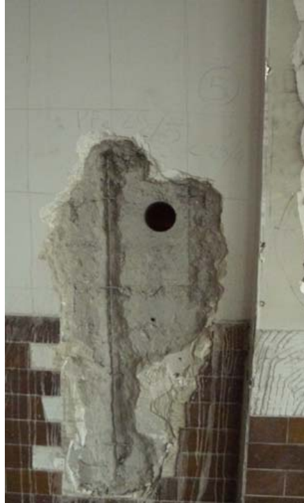
Figure 3. Survey after pachometer investigation.
