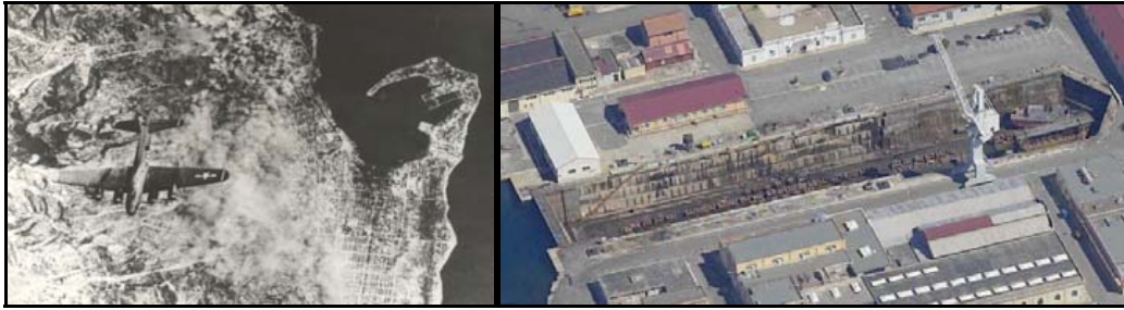
Figure 2. Aerial view of Messina with the identification of the port (left) and of the dry dock within the port (right)
